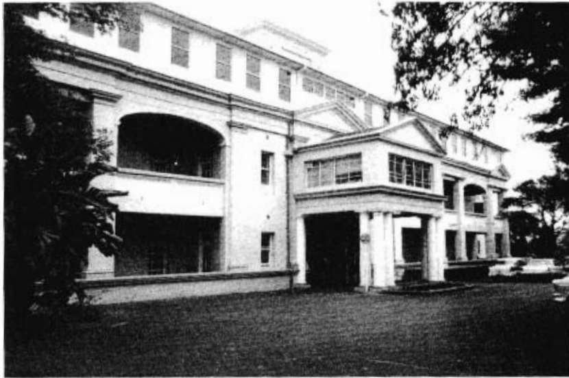
N.S.W. Masonic Hospital, Ashfield Refer page 419.
