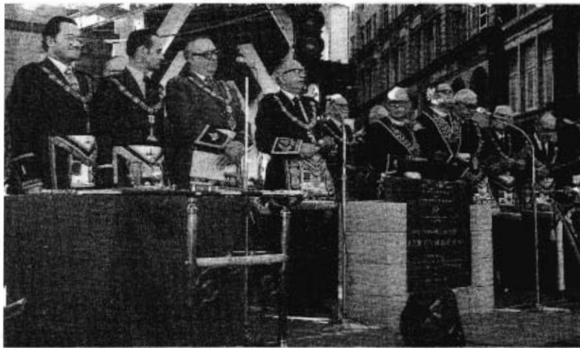
Setting the Foundation Stone, Memorial Masonic Centre, Sydney Refer page 317.
